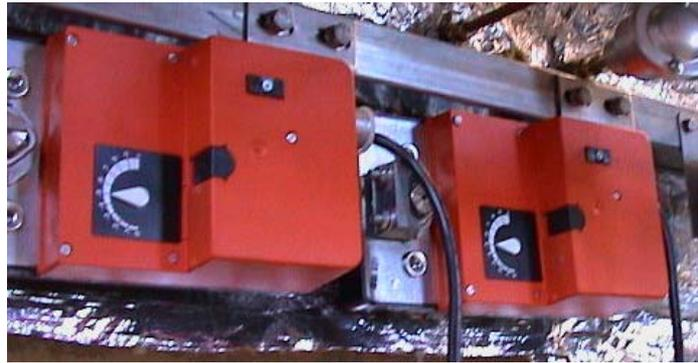
Figure 3.2 Servo motors for valves
