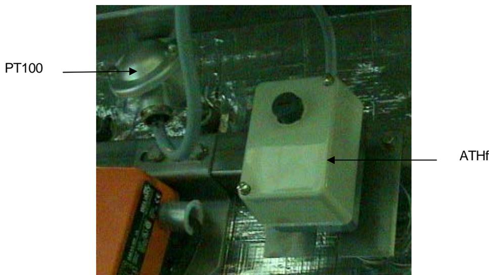
Figure 3.6 PT 100 and maximum thermostat
